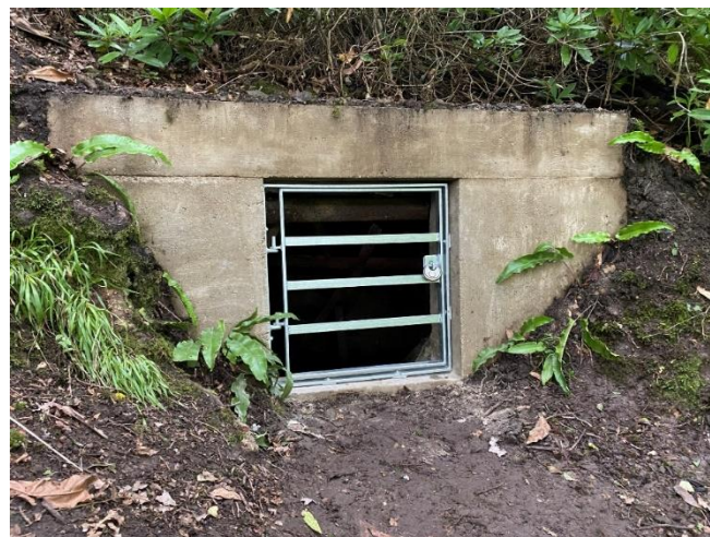
Completed repairs to small hibernation site, South Wiltshire © G. Harris
